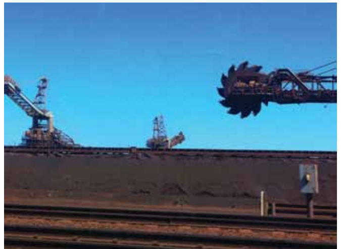
Reclaimer at Cape Lambert moving the stockpiles of iron ore
