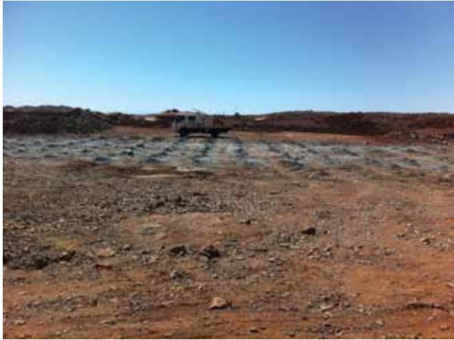
Ground being prepared for blasting at Cape Lambert
